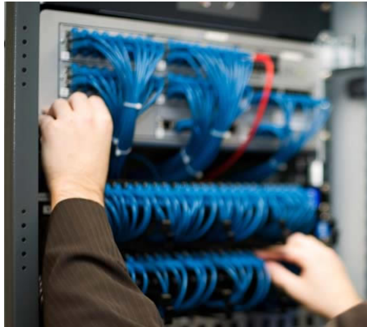
You might spend hours on cable dressing, but the benefits are worth it.
